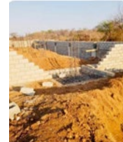
COMPLETION OF COLUMN BASES REINFORCEMENT AND PLACEMENT IN READINESS FOR CONCRETE POURING
