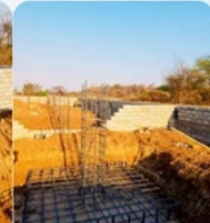
COMPLETION OF COLUMN BASES REINFORCEMENT AND PLACEMENT IN READINESS FOR CONCRETE POURING
