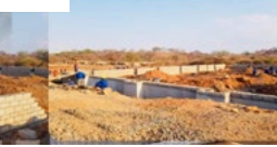
CONSTRUCTION OF INTERIOR FOUNDATION WALLS IN READINESS FOR BACKFILLING & COMPACTION
