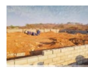
CONSTRUCTION OF INTERIOR FOUNDATION WALLS IN READINESS FOR BACKFILLING & COMPACTION
