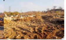
EARTH MOVING TO THE MAIN ENTRANCE IN READINESS FOR BACKFILLING
